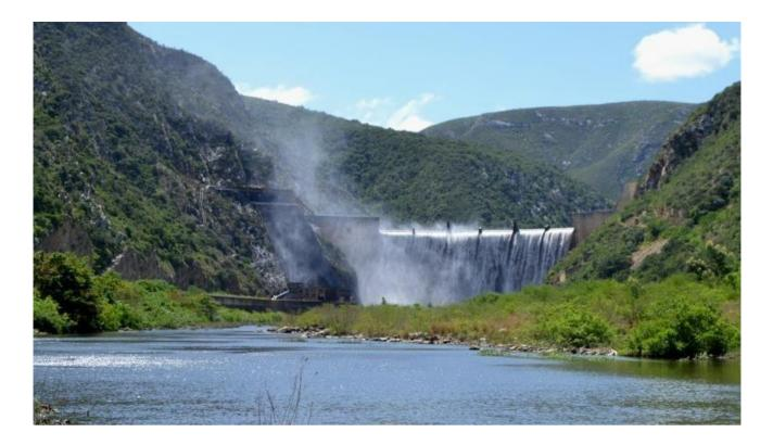
Figure 10. Typical concrete gravity dam spillway, allowing overflow descending over the middle part of the dam crest
